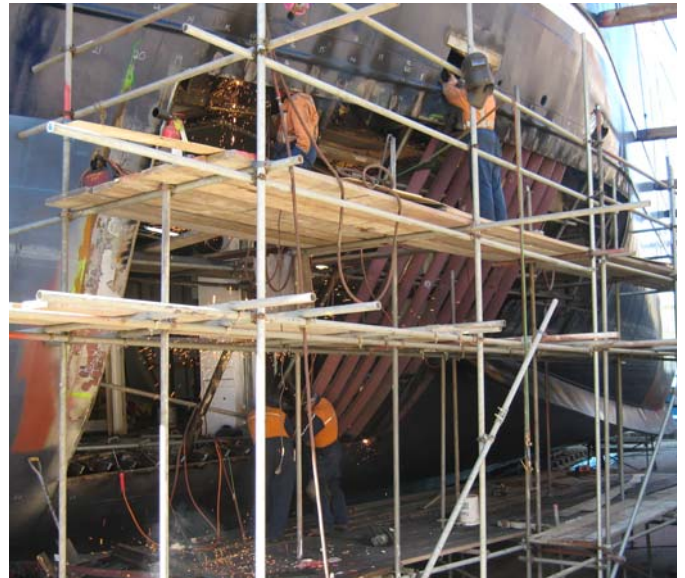
San Aspiring – Hull Plate Replacement
