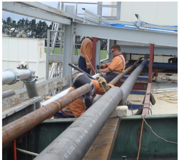
Pipe work installation – Talley's Foods Ashburton
