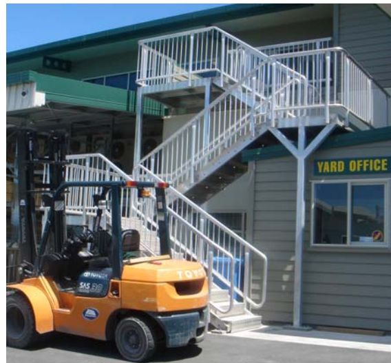
Guardway stairs – Kaikoura timber plant
