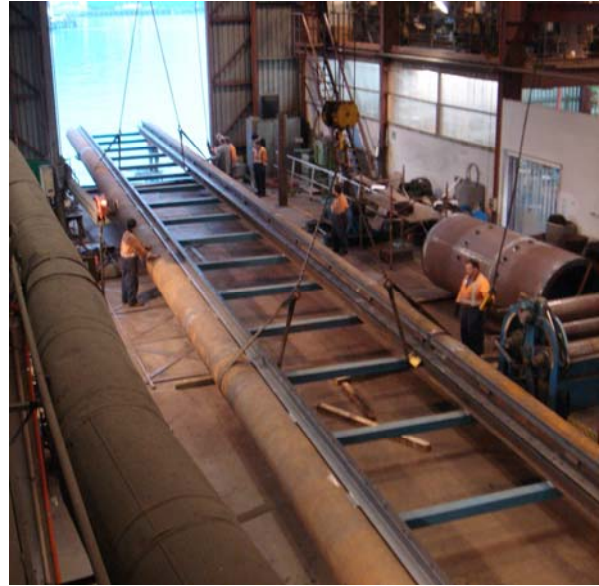
Pipe launching raft – Waste water ocean outfall
