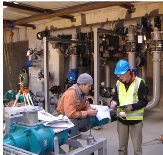
Pipework installation – Bromley waste water plant
