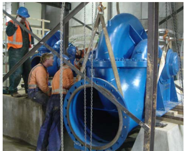
Pump installation – Black Point Irrigation Scheme
