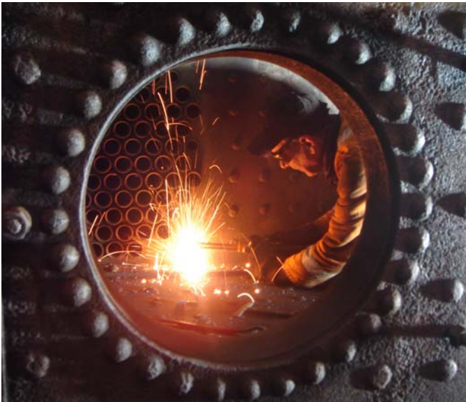
Firebox repairs – Price V locomotive boiler
