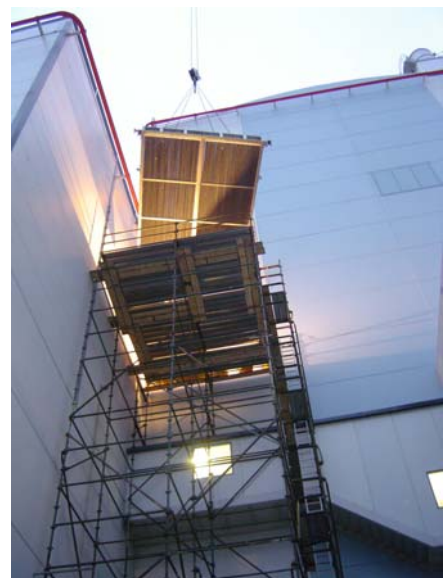
Dryer installation – Clandeboye Plant
