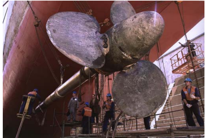
Prop Shaft Repairs – Malakov Kurgan
